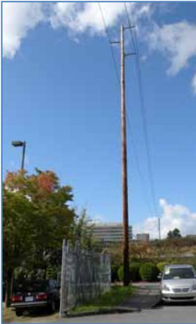
Example pole with average heights ranging from 65 feet to 75 feet depending on topography and span length.
