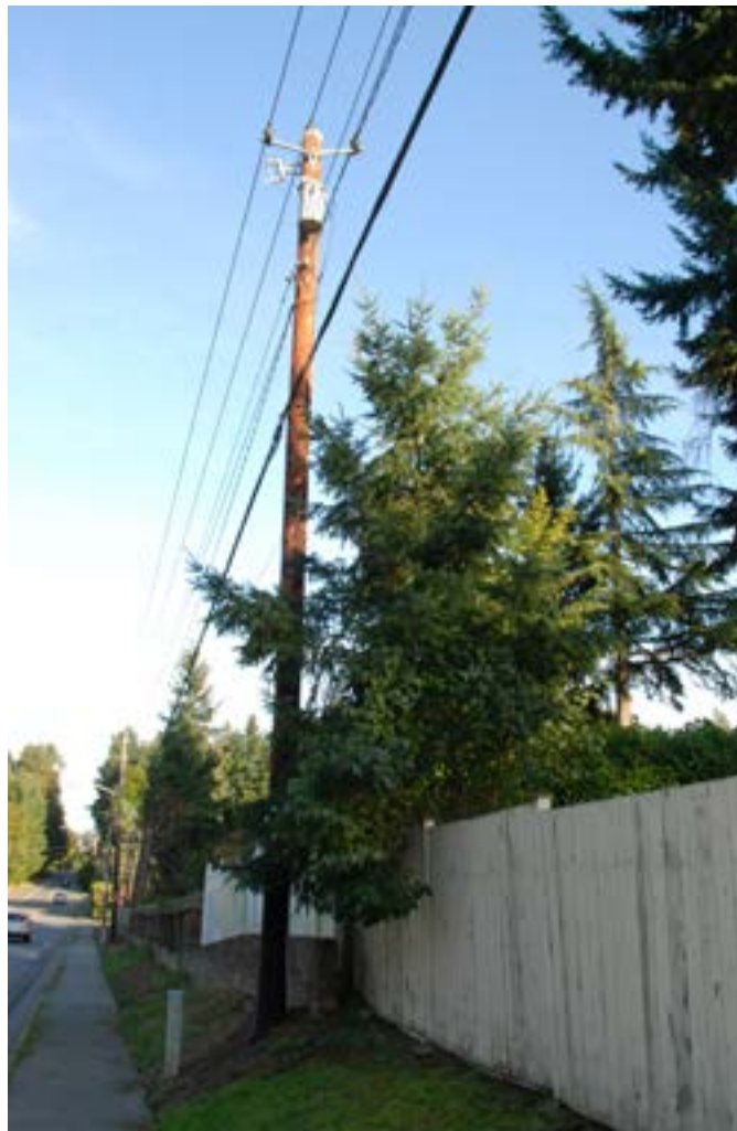
Three Phase Distribution – Compact Construction
