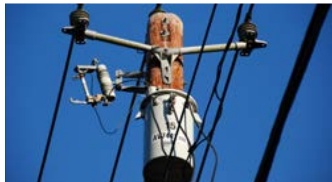
Three Phase Distribution – Compact Construction
