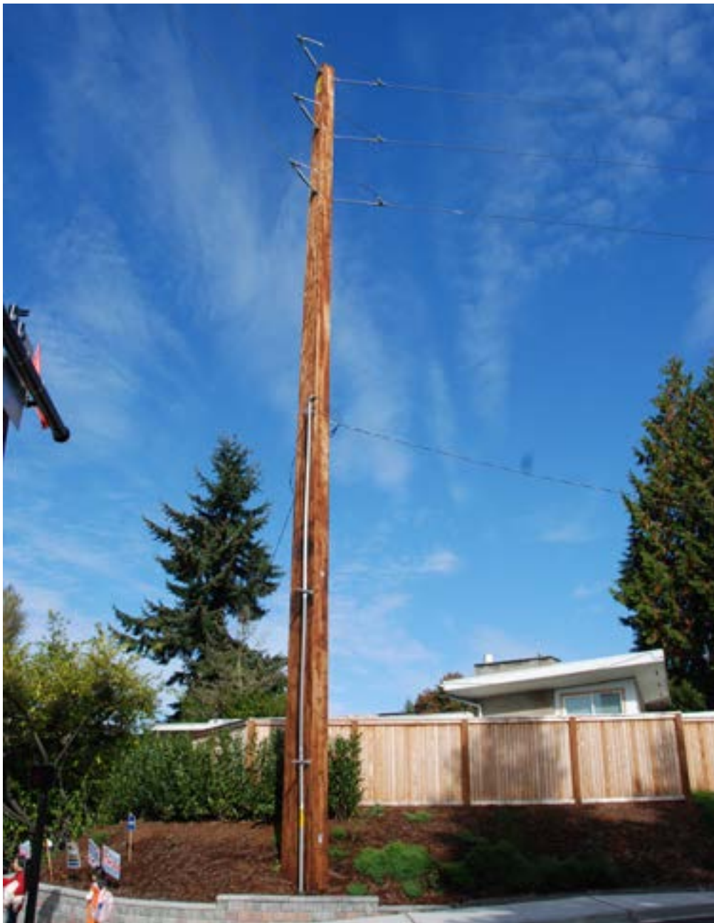
Typical 115kV Transmission Pole Glu-lam (laminated wood rectangular)
