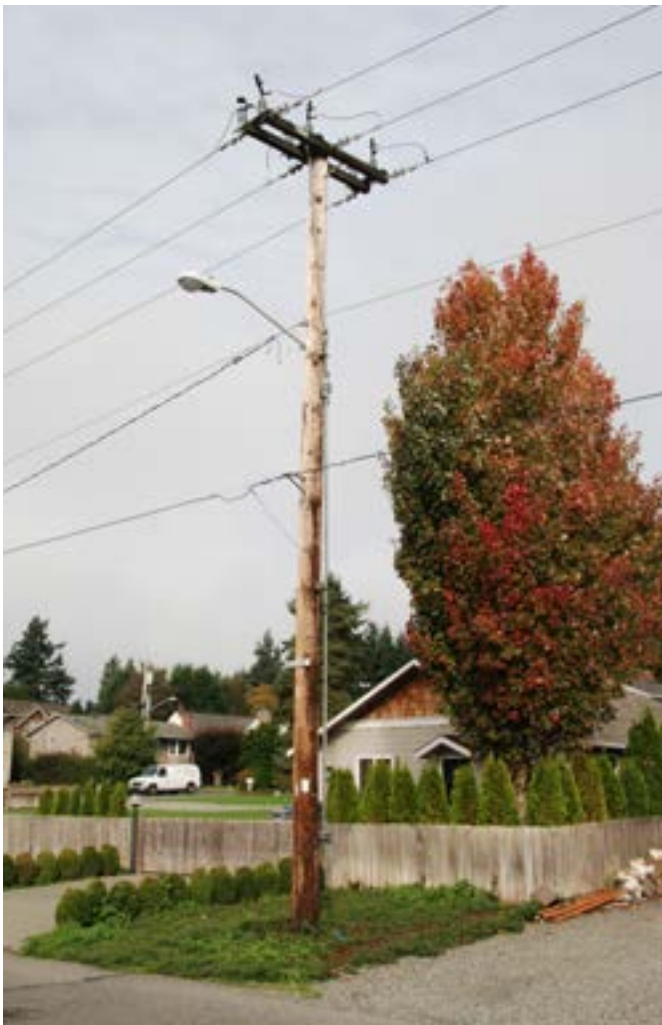
Three Phase Distribution with Gang Operated Switch
