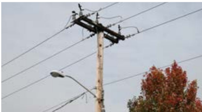
Three Phase Distribution with Gang Operated Switch
