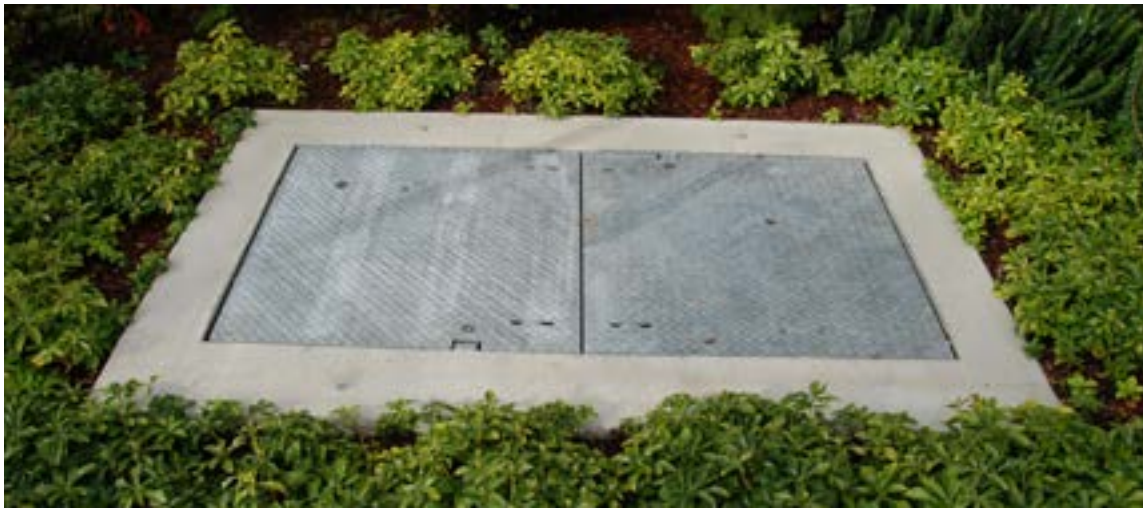
Typical Underground Distribution Cable Junction Vault (5' X 7')
