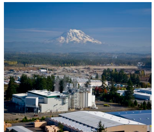
▲ Frederickson 1 Generating Station
