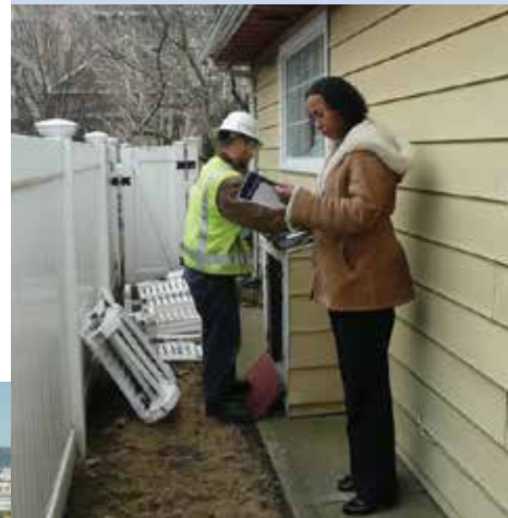
Brandon Severson, PSE customer service field technician who operates in Seattle, inspects a New York City homeowner's natural gas service that was damaged by flood water.
