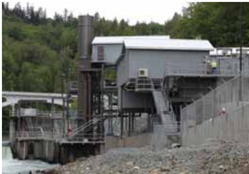
PSE’s new Baker River fish trap-and-haul facility
