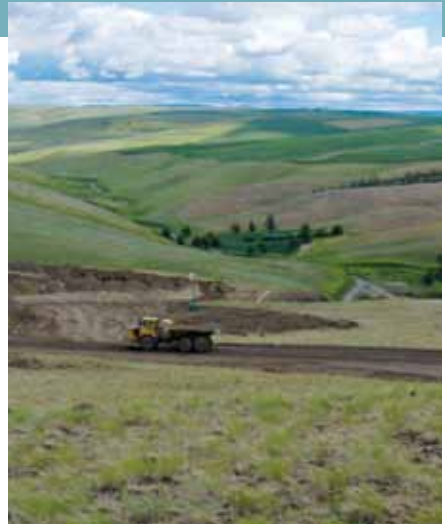
Grading roads for the project
